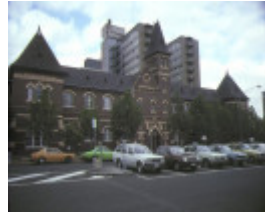
1 former faraday street primary school carlton front elevation feb1985
