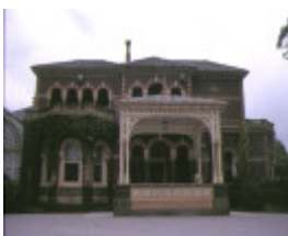
1 ripponlea elsternwick front entrance
