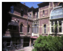
ripponlea elsternwick service wing & yard nov1984
