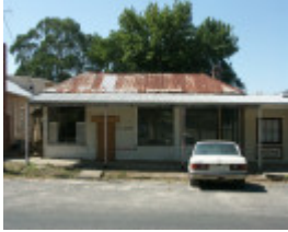
Shop (east shop of pair)
