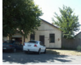
Shop (east shop of pair)
