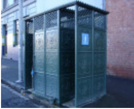
Urinal Queensberry & Elizabeth St exterior KJ 21 06 2007
