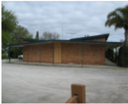
Oakleigh Motel_eastern block_KJ_Sept 08
