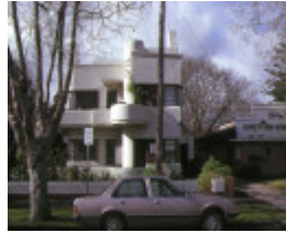
1 windermere flats broadway elwood front elevation jul1989
