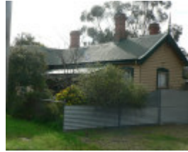
Former Police Station and Residence, 42 Ferrars Street Rokewood
