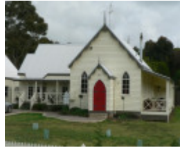
Former Presbyterian Church, 143 Russells Bridge Road, Russells Bridge
