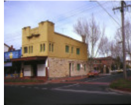
1 former chemist shop ormond road elwood front view
