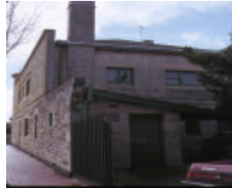
former chemist shop ormond road elwood rear view
