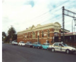
Caulfield Railway Station platform 4, August 1995
