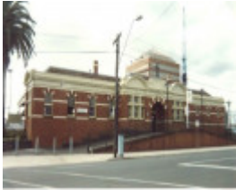
Caulfield Railway Station, platform 1, August 1995
