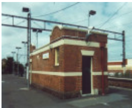
Caulfield Railway Station stores building, August 1995
