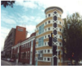
Cnr Railway Avenue and Dandenong Rd, August 1994
