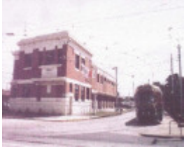
Glen Huntly Tram depot, Glen Huntly Rd Caulfield
