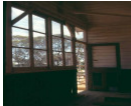
h02051 natimuk primary pavilion interior2
