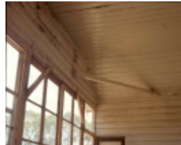
h02051 natimuk primary pavilion interior
