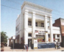
State Savings Bank 438 Centre Rd Bentleigh
