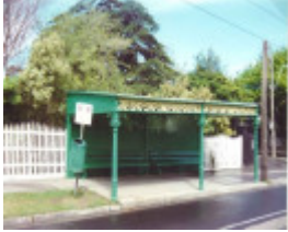
Tram Shelter Corner Balaclava & Orrong Roads Caulfield
