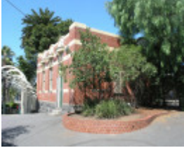
ESSENDON RAILWAY STATION COMPLEX SOHE 2008
