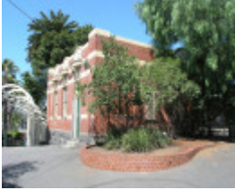
ESSENDON RAILWAY STATION COMPLEX SOHE 2008
