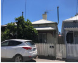
9 Bayview Street, Prahran
