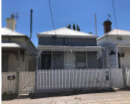
11 Bayview Street, Prahran
