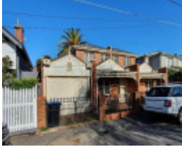
34-36 Bayview Street, Prahran
