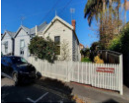
58-60 Bayview Street, Prahran
