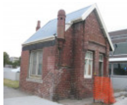
Former Ferry Terra Cotta & enamel brickworks office albert Street brunswick from the northwest
