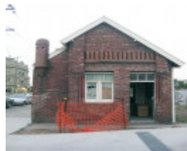
Former Ferry Terra Cotta & enamel brickworks office albert Street brunswick west facade with door open
