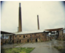
Former Ferry Terra Cotta & Enamelled Brickworks Office Albert Street Brunswick Kiln 1997
