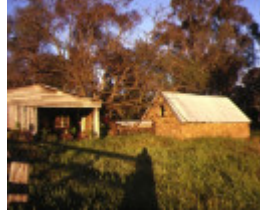
stone cellar at faithfuls creek hume hwy euroa view of property prior to damage
