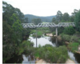
TIMBER TRUSS AND CONCRETE BRIDGE SOHE 2008
