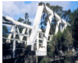
h01214 timber truss and concrete bridge over genoa river genoa northern end she project 2003
