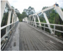
TIMBER TRUSS AND CONCRETE BRIDGE SOHE 2008
