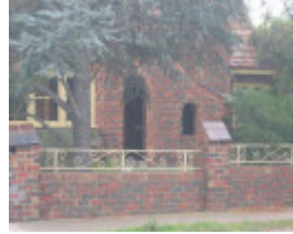
18 Barton Street, Fence
