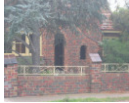
18 Barton Street, Fence
