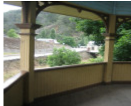
Walhalla Bandstand looking towards stone wall
