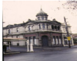
1 former kensington property exchange office shop & residences bellair street kensington front view apr1996
