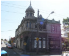
FORMER KENSINGTON PROPERTY EXCHANGE, OFFICE, SHOP AND RESIDENCES SOHE 2008
