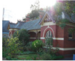
4435 Royal Freemasons Homes 313 Punt Road Building 02
