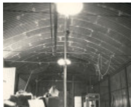
Porter prefabricated iron store
