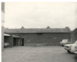
Porter prefabricated iron store
