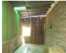
Former Exford Shearing Shed
