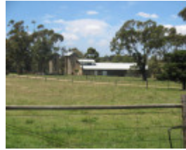
Former Exford Shearing Shed
