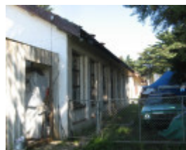
Beam Wireless Receiving Station Mt Cottrell side of operations building
