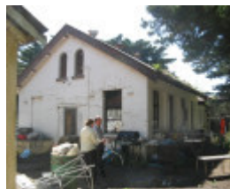
Beam Wireless Receiving Station Mt Cottrell operations buildings from west
