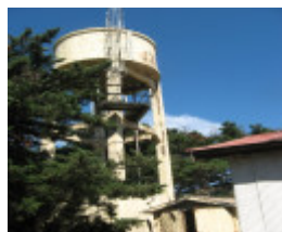
Concrete water tower
