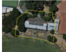
Extent of registration aerial
