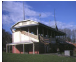
fitzroy cricket ground grandstand brunswick street fitzroy side view aug1985
