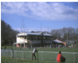
fitzroy cricket ground grandstand brunswick street fitzroy site view
