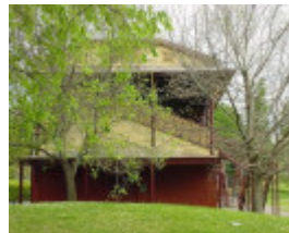
h00751 fitzroy cricket ground grandstand brunswick street fitzroy side view she project 2004
