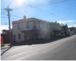
Plenty Road Commercial Precinct
