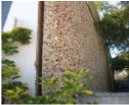
Former Shire Offices_Benalla_aggregate wall_KJ_5/9/08
