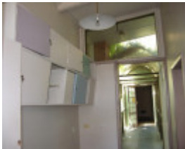
Former Benalla Shire Offices_kitchen cupboards_KJ_Sept 08
