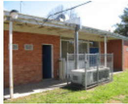
Former Benalla Shire Offices_rear wall_KJ_Sept 08
