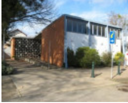
Former Shire Offices_Benalla_JC_Aug 08
