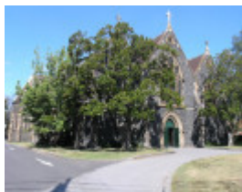
ALL SAINTS CHURCH, HALL AND FORMER VICARAGE SOHE 2008
