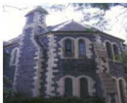
1 all saints church hall & former vicarage chapel street east st kilda rear view of church may1997
