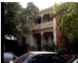
St Marks George St Fitzroy Vicarage
