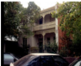
St Marks George St Fitzroy Vicarage
