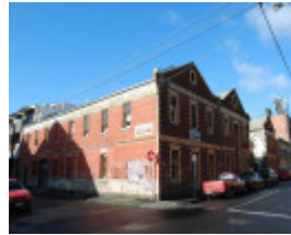
4555 Former Cordial Factory View South East 10
