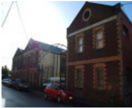
4555 Former Cordial Factory View North East 10
