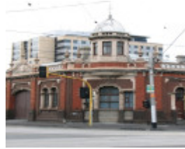
FORMER CABLE TRAM ENGINE HOUSE SOHE 2008
