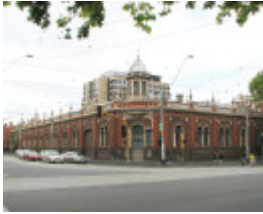
FORMER CABLE TRAM ENGINE HOUSE SOHE 2008
