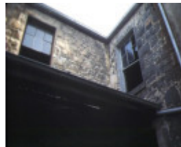
glass terrace gertrude street fitzroy rear stonework aug1978
