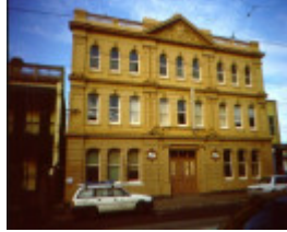
H01967 1cathedral hall facade
