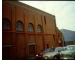
H01967 cathedral hall south elevation
