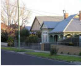
45831 McKay Housing Estate - Durham Rd
