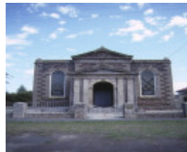
Former Wesleyan Church Parsonage & Common School James Street Port Fairy Front View of Church February 1990
