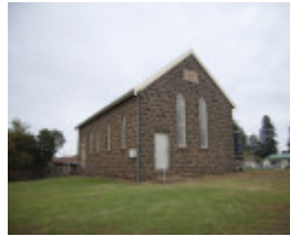
FORMER WESLEYAN CHURCH, PARSONAGE AND COMMON SCHOOL SOHE 2008
