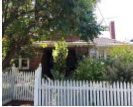
77 Stanhope Street, Malvern
