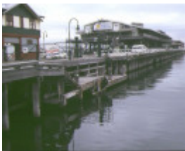
1 station pier port melbourne side view of pier
