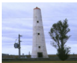
1 leading lights beach road port melbourne view of inner leading light
