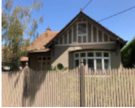
80 Stanhope Street, Malvern
