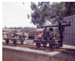
h00993 torrumbarry weir lock chamber steam boiler and steam winch complex torrumbarry drop bar hydraulic operated she project 2004
