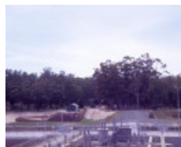
h00993 torrumbarry weir lock chamber steam boiler and steam winch complex torrumbarry view of site she project 2004
