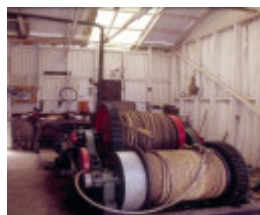
h00993 torrumbarry weir lock chamber steam boiler and steam winch complex torrumbarry winch house interior she project 2004
