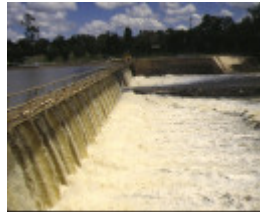
1 torrumbarry weir complex face of weir
