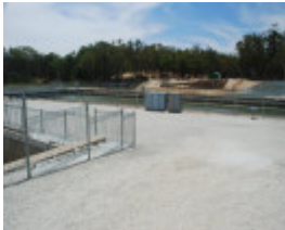
TORRUMBARRY WEIR LOCK CHAMBER, STEAM BOILER AND STEAM WINCH COMPLEX SOHE 2008
