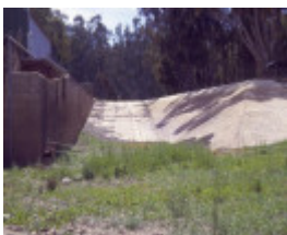
h00993 torrumbarry weir lock chamber steam boiler and steam winch complex torrumbarry trestle runway she project 2004
