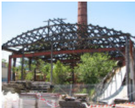
WUNDERLICH/MONIER TERRACOTTA ROOF TILES COMPLEX SOHE 2008
