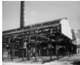
1 wunderlich terra cotta tile works demolished mitcam road vermont view structure
