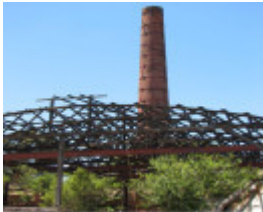
WUNDERLICH/MONIER TERRACOTTA ROOF TILES COMPLEX SOHE 2008
