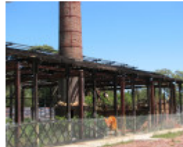
WUNDERLICH/MONIER TERRACOTTA ROOF TILES COMPLEX SOHE 2008
