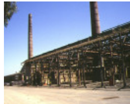
1 wunderlich terra cotta tile works demolished mitcam road vermont view of chimneys nov1993
