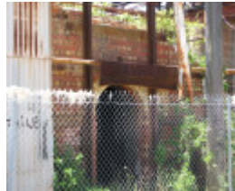
WUNDERLICH/MONIER TERRACOTTA ROOF TILES COMPLEX SOHE 2008
