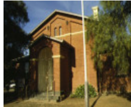
1 flormer pleasant creek court house longfield street stawell front view
