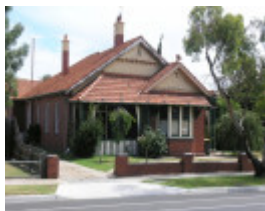
FORMER MANAGER'S RESIDENCE, NEWPORT RAILWAY WORKSHOPS SOHE 2008
