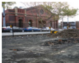
H0988 former cable tramway engine house tracks2 abbotsford may2007 street north melbourne
